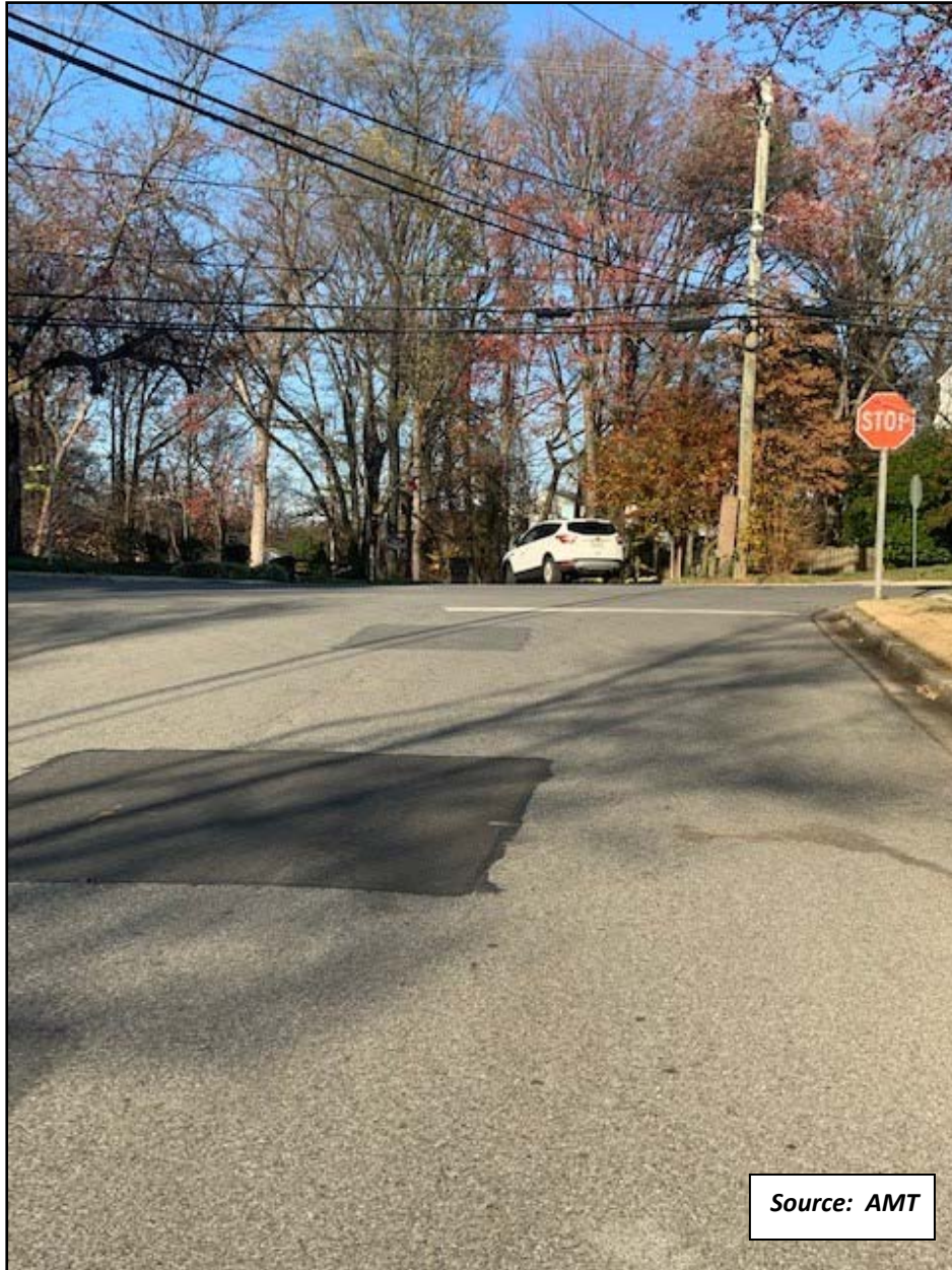
Crest Avenue – Looking North
