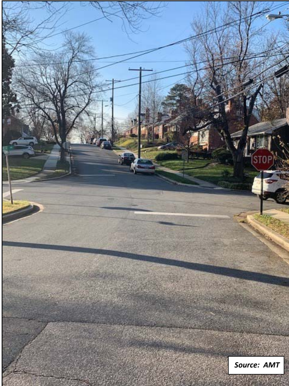
Lockwood Road – Looking West
