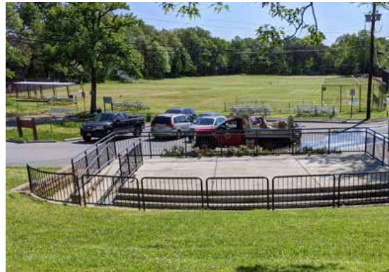
No permanent seating around amphitheater
