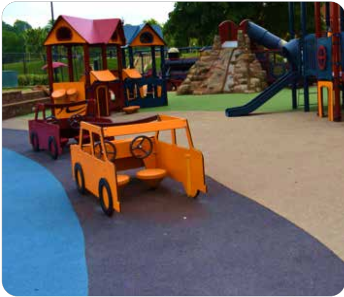
Permeable rubber playground surface with subsurface water storage
