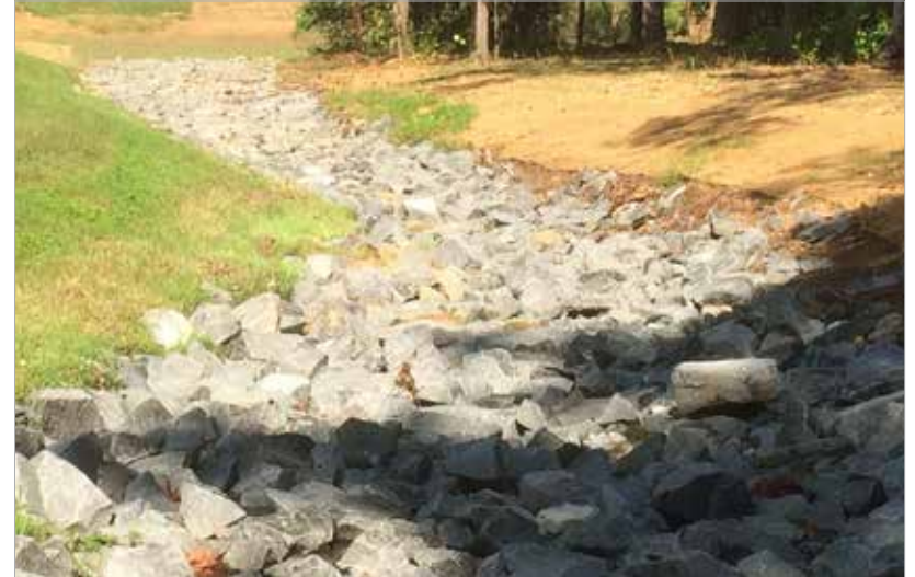
A channel stabilized with rock/riprap
