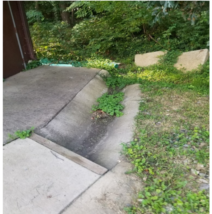
Concrete Channel on the South
