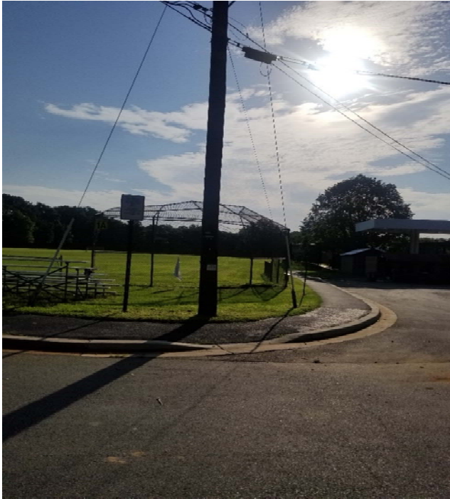
Onsite Power Pole at Park Access Trail
