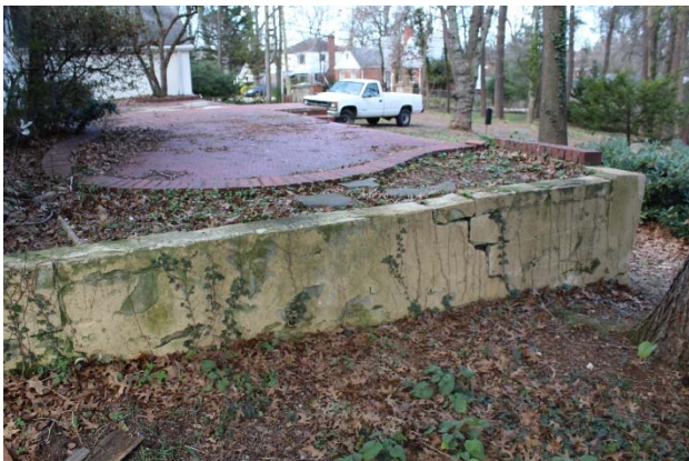
Photo 24- Damages to side of front patio foundation wall
