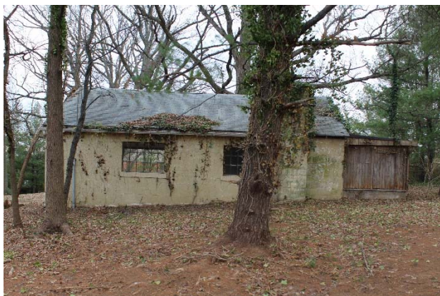
Photo 18- West side of storage garage. Pointing required. Rear wooded shed should be demoed
