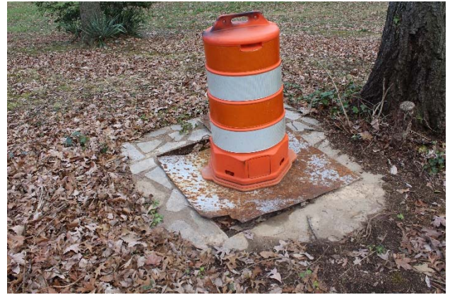
Photo 13- Unsecured storm drain access needs to be addressed
