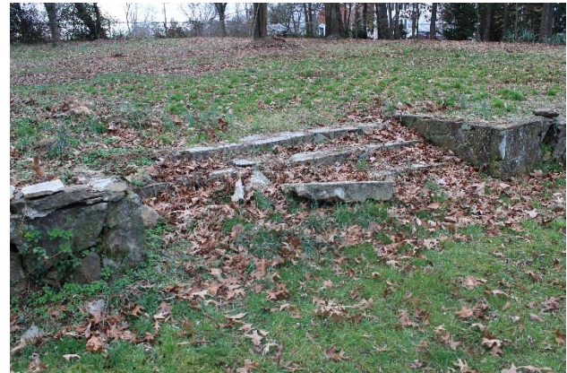
Photo 7- Damaged steps of rear landscape retaining wall
