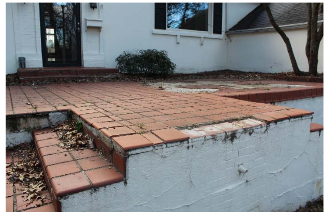
Photo 25- Damages to front patio and steps tile work & slab. Also a code issue since there is not guardrail or handrails.
