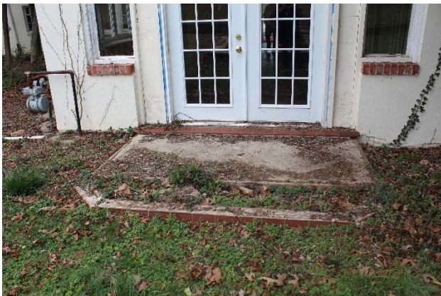
Photo 29- Damages to landing pad from Parlor room.
