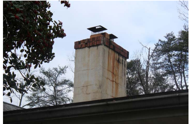
Photo 28- Chimney needs repair of cracks, stains, tilework.
