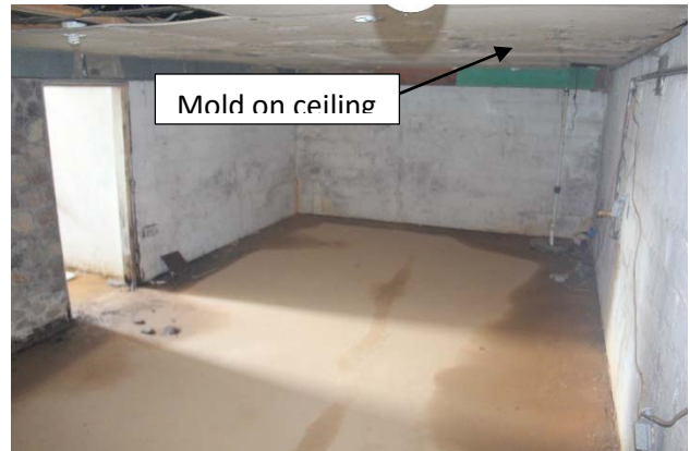
Photo 38- Basement. Wet slab can be sign of sump pump failure. Mold on ceiling and walls
