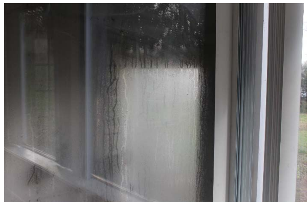
Photo 36- Window condensation on interior Bedrm window
