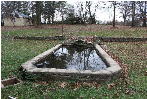
Photo 8- Pond w/ filtering control inset on left. Pointing needed
