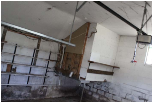
Photo 41- Sample interior view of garage. Wet slab, pointing needed, mudroom/laundry rm extension is not structurally sound. Needs to be removed.
