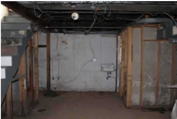
Photo 39- Basement. Mold on walls, wet slab, and non-structurally sound stairs
